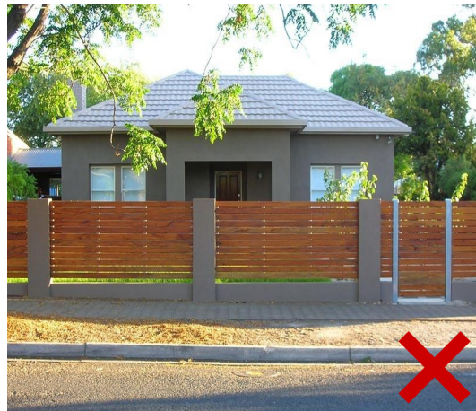
(The fence is located within the front setback area and is also above 3 feet in height)
